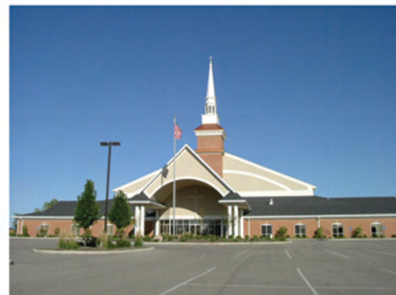
Urbancrest Baptist Church, Lebanon, OH
